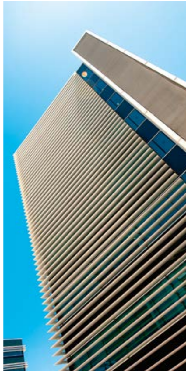
OFFICE PARK EXPO, Lisbon (Portugal)
